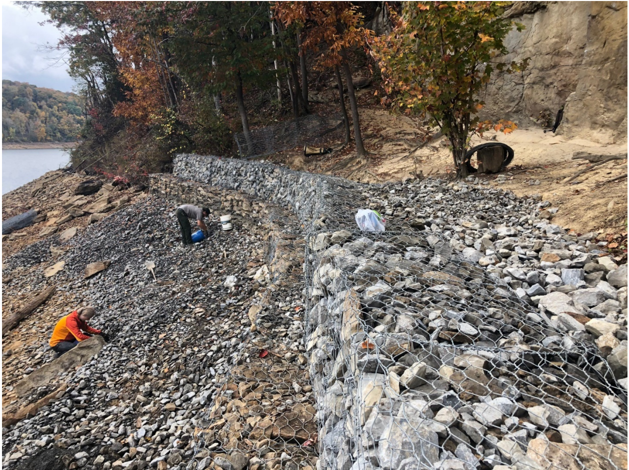
The first row of baskets being assembled at Orange Oswald.
