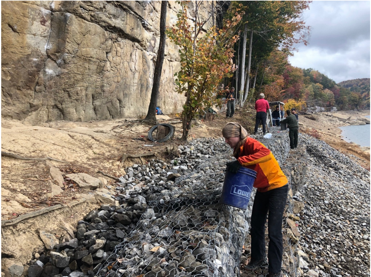
A volunteer from the New River Alliance of Climbers readies to pour a bucket of rocks behind the newly constructed gabion baskets.
